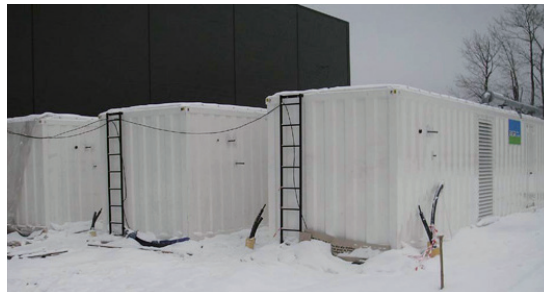
The Algerian state power company 20 units, 880KVA, 10KV container rites high voltage gensets runs weaver.
