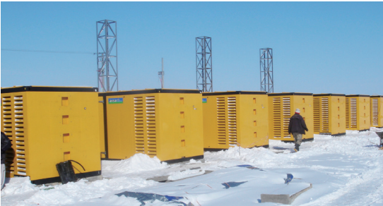
The Algerian state power company 20 units, 880KVA, 10KV container rites high voltage gensets runs weaver.
