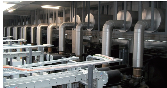
British Tesco supermarket, 31 units gensets, power involves 650KVA~1435KVA, the total capacity of 34065KVA.
