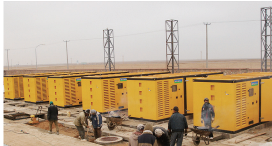
The Algerian state power company 20 units, 880KVA, 10KV container rites high voltage gensets runs weaver.
